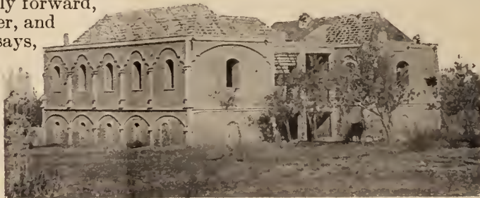
LILY REID HOLT MEMORIAL HOSPITAL at Hamadan, Persia; completed in 1907. J. A. Funk, M.D., in charge.
